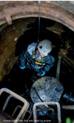
wastewater on into the sewer system on the way to the treatment plant. Photo: Fredericia Spildevand og Energi
